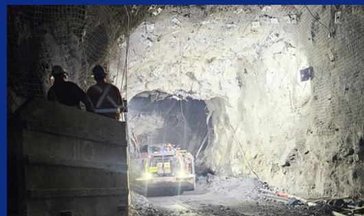
A crew removes more than ~2,500 tonnes of material from the decline using manual and remote-controlled scoops.
